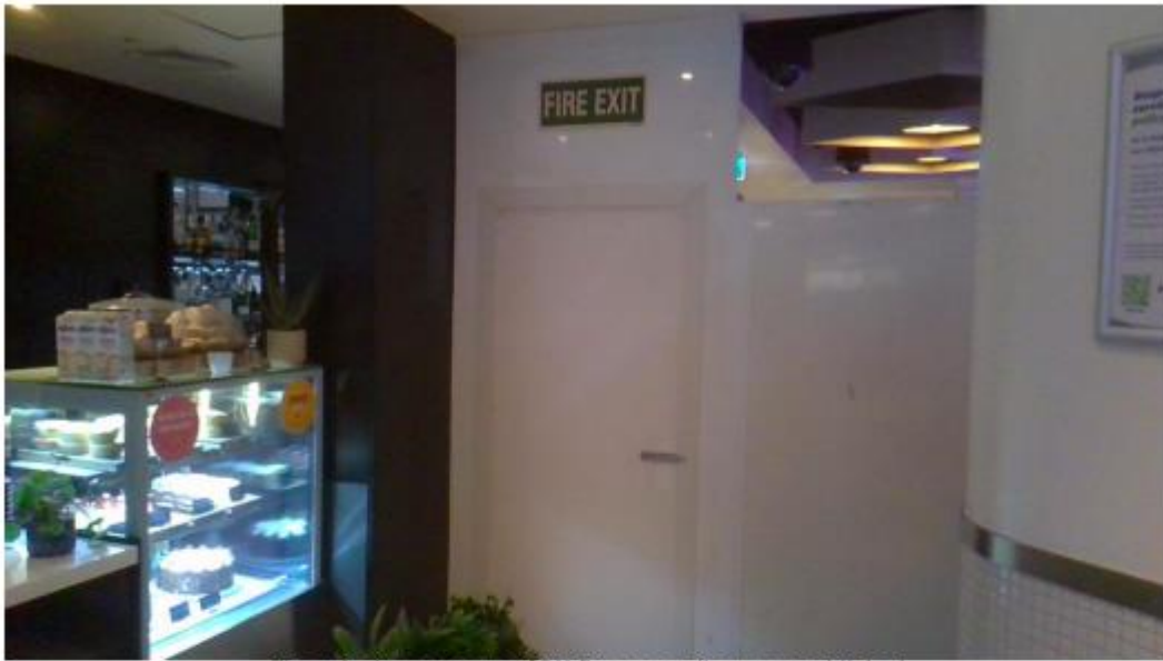
Fire exit signage as per CPU fire report diagram established Taken at 11:16 AM on Tuesday 15/04/2025
